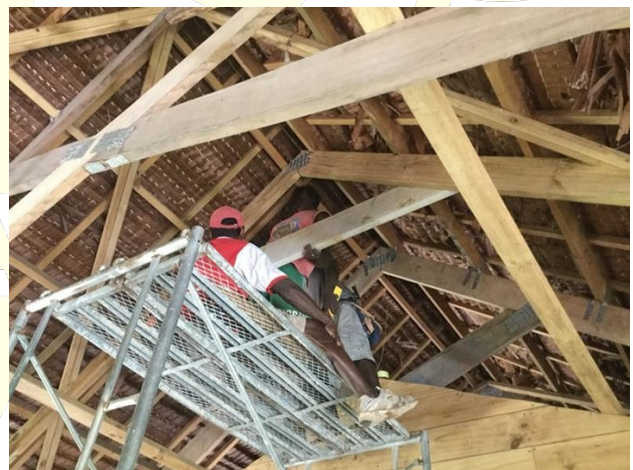
New trusses being placed on the existing building as reinforcements for the new colour bond application.
